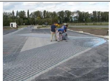
Right: fixing of pipes (© REHAU)
